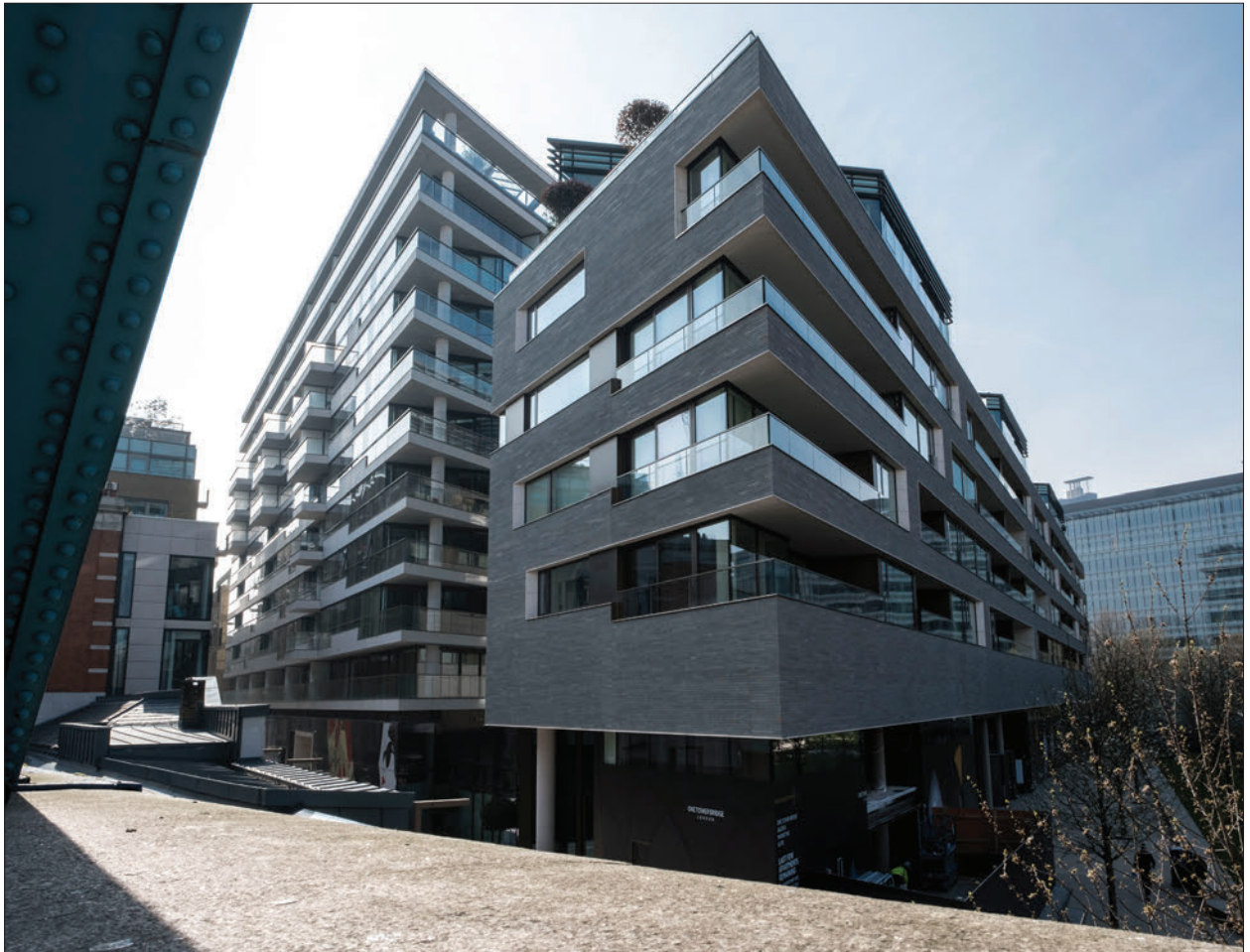
One Tower Bridge, Southwark
