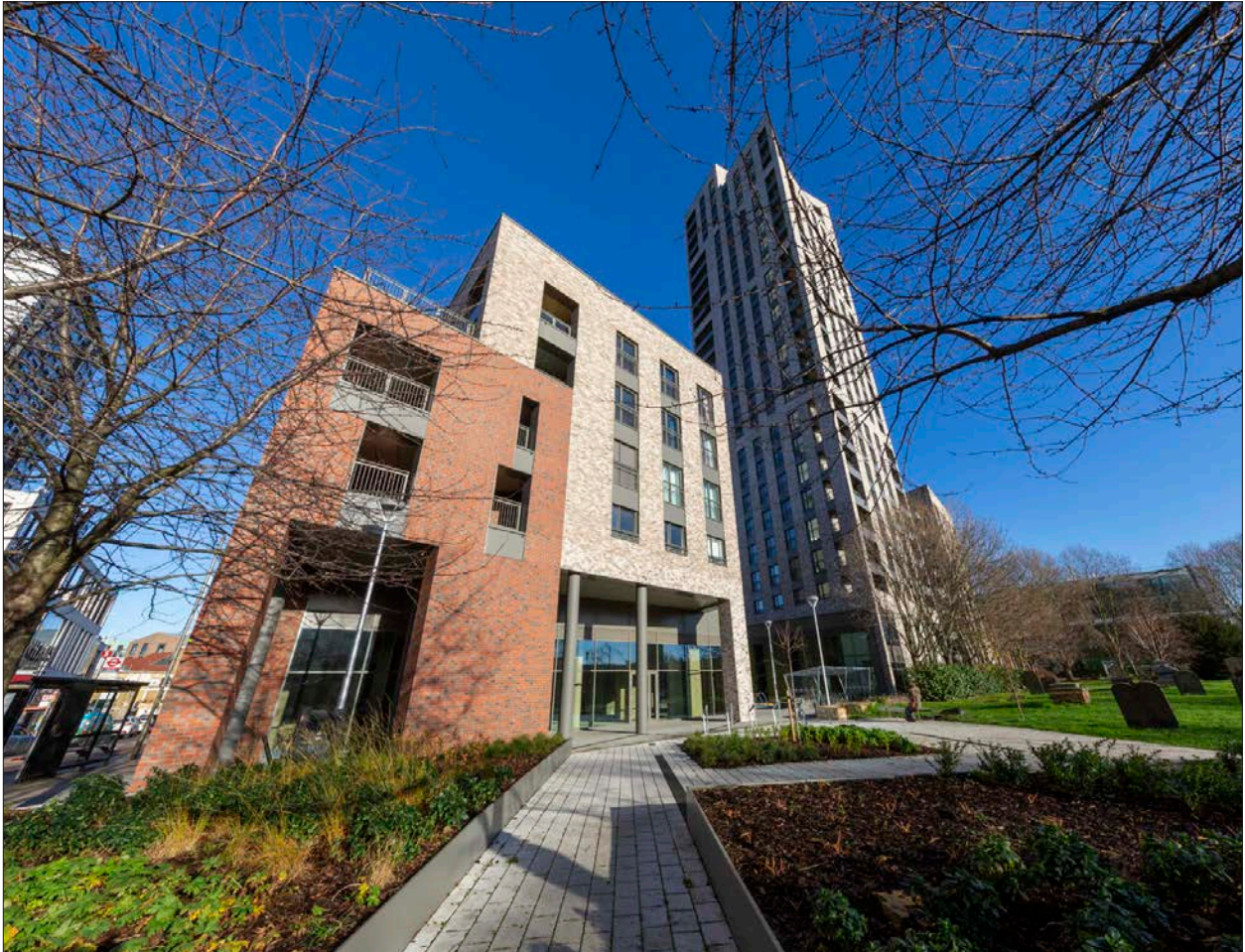
Wandsworth Exchange, Wandsworth
